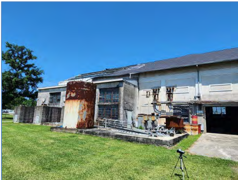
Figure 3.2: Exterior of Old Diesel Plant
