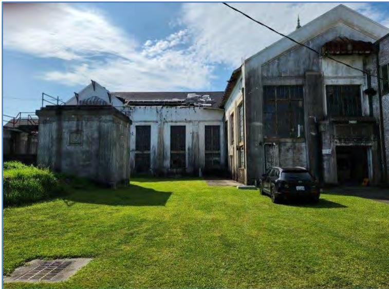
Figure 3.1: Exterior of Old Diesel Plant
